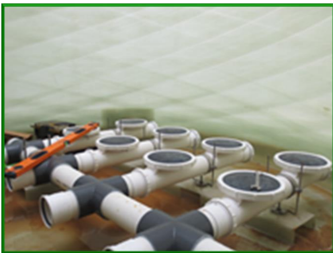
Figure 9.27. Semi-industrial plant for the treatment of 20 m 3 /day of leachate, developed under the project Advanced LFT.
