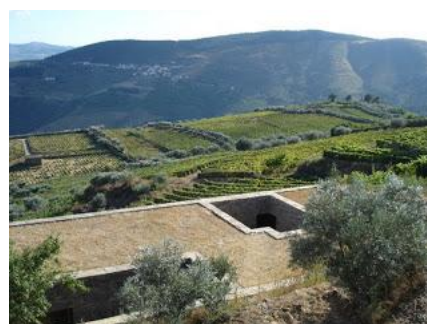
Figure 39 House in Provesende. Green roof (Ramos 2007)
