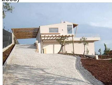
Figure 35 Óasis House. West façade (Nascimento and Gonçalves 2005)
