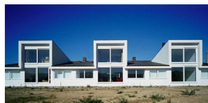
Figure 37 Houses in Janas. South façade (Mourão and Santa Rita 2003)
