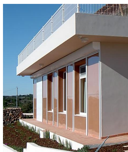
Figure 36 Óasis House. Thermal storage wall (Nascimento and Gonçalves 2005)
