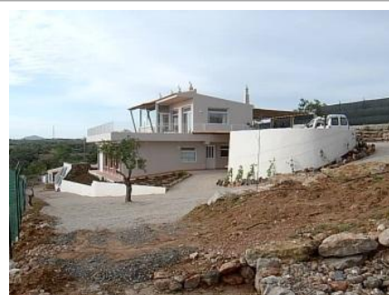
Figure 34 Óasis House. East façade (Nascimento and Gonçalves 2005)
