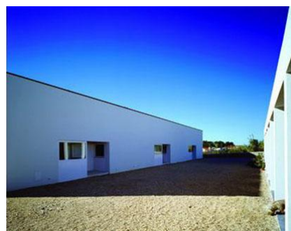
Figure 38 Houses in Janas. North façade (Mourão and Santa Rita 2003)
