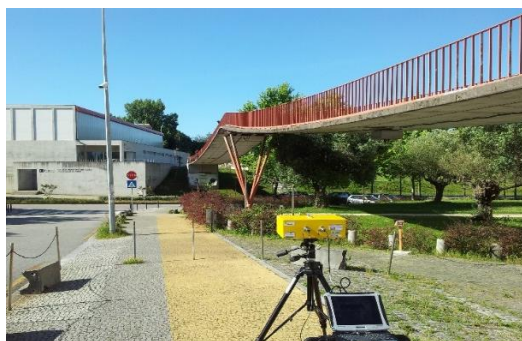
Fig. 6.44 - Ponte Pedonal FEUP
