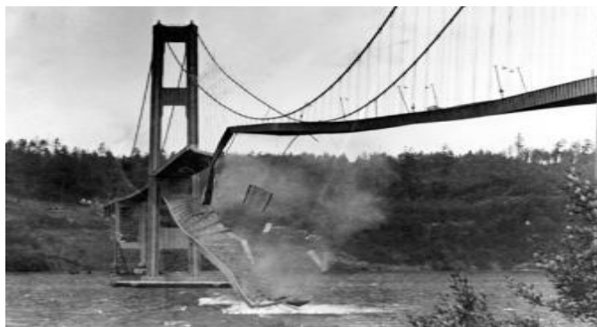
Fig. 2.2 – Colapso da ponte Tacoma Narrows Bridge [17]
