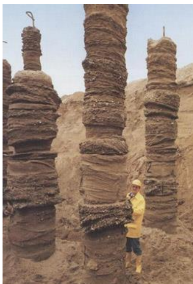
Figura 4.4 - Colunas de jet-grouting (Bilfinger Berger Foundations)
