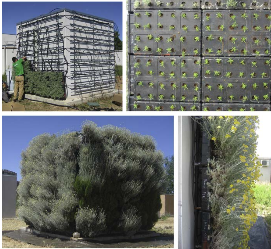
Figure 27 - Green Wall made with polyethylene modules, coconut fibre substrate and native shrubs. (Pérez, et al., 2016)
