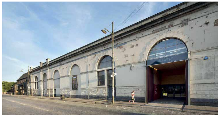
Figura 209 - Entrada do Tramway Theatre, 2016
