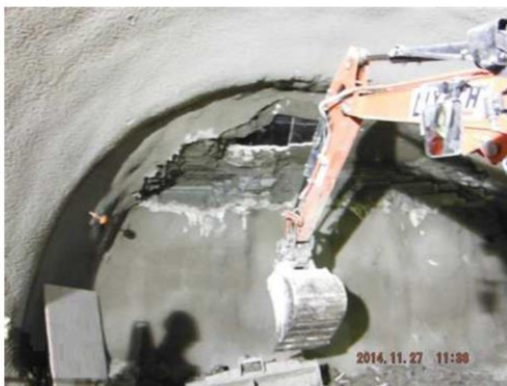
Figure 4.10 - Construction of the underpass: exposing the POT cast iron lining (HAT courtesy)
