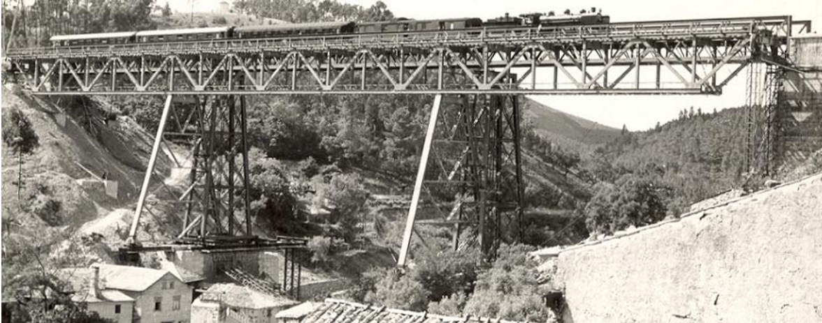
Figure 2.6 – The old and new Trezói bridge (1956)
