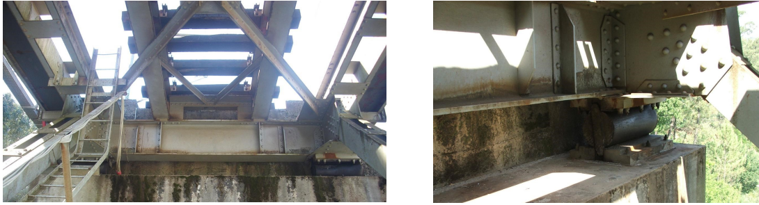
Figure 5.3 – Local view of the cross-girder at the end support.
