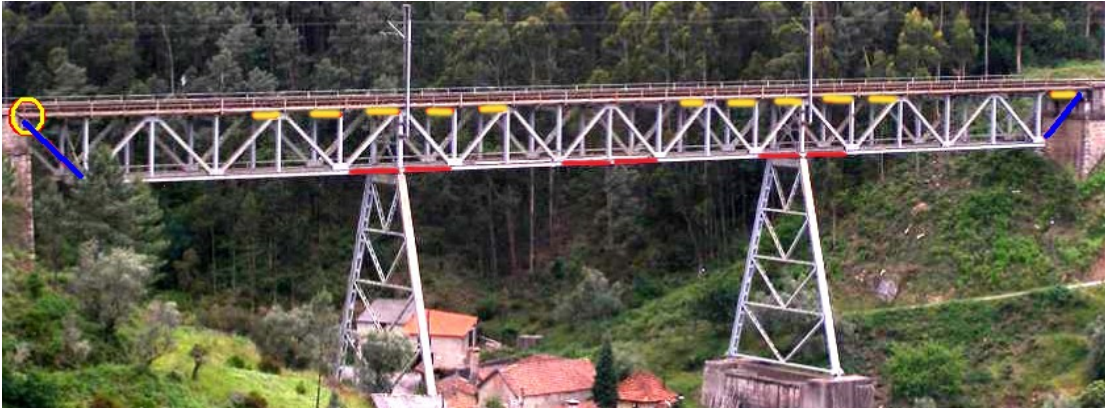
Figure 5.53 – Characterization of the elements more affected by fatigue according to the global fatigue assessment results using a bar FEM (yellow – cross-girders; blue – diagonals; red – bottom chords)
