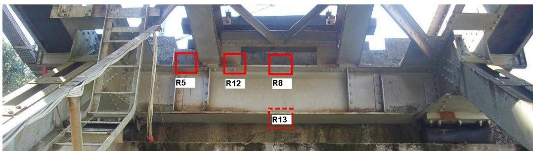
Figure 5.12 – Locations of the accelerometers at the extremity cross-girder.
