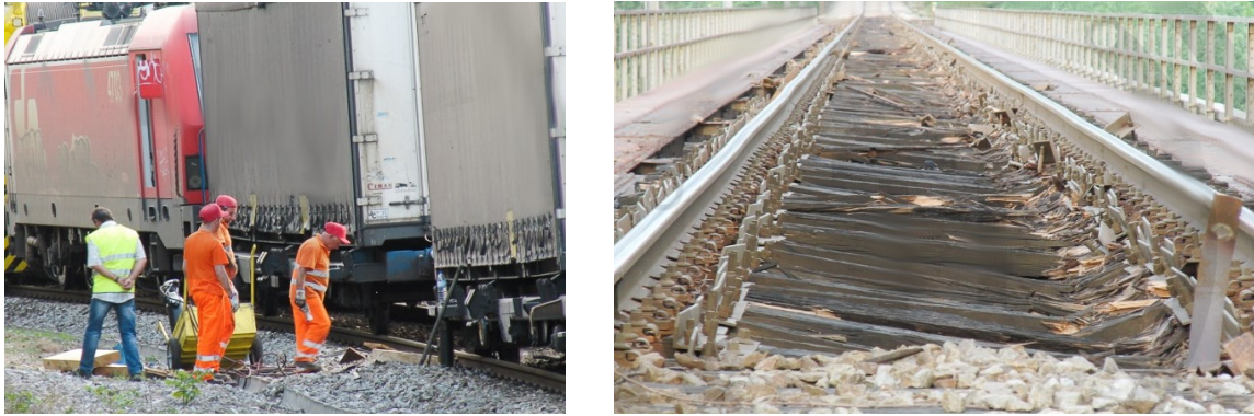
Figure 5.47 – Derailed train and the consequences on the railway
