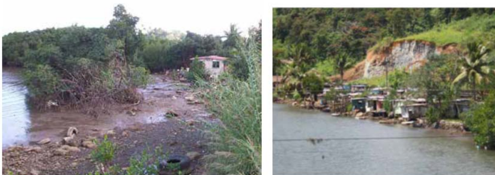
Figure 25: Squatter settlements on vulnerable areas
