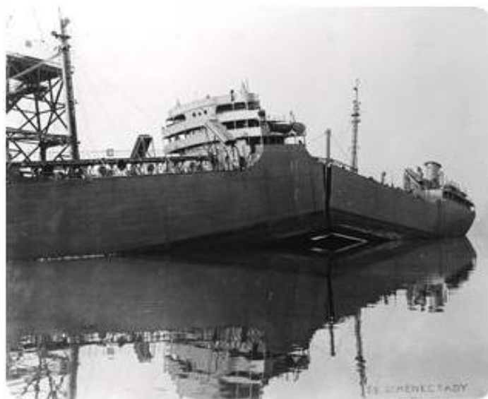
Figure 2.2 - Brittle fracture of a vessel due to unstable propagation of fatigue cracks (Hayes, 1996).
