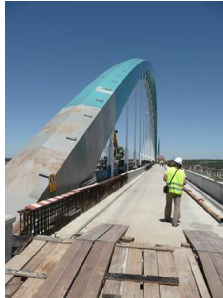
Figure 6.31 - Concreting of a ballast-guard.
