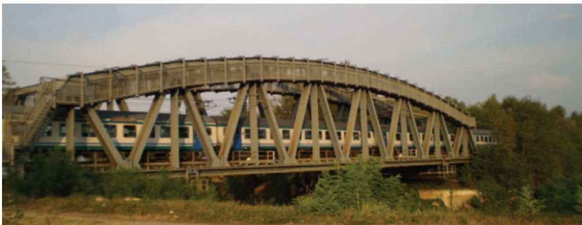
Figure 2.31 – Panaro Bridge (Lippi et al., 2011).
