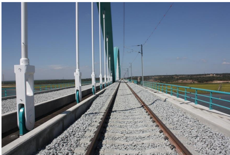
Figure 6.17 - Ballasted track located at the upstream side of the bridge.
