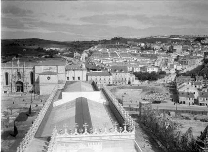
Figure 5. The Affordable Houses Neighbourhood of Belém behind the Monastery of Jeronimos, Lisbon, 1938-39. Construction works for the Portuguese World Exhibition of 1940 are visible on the bottom right. (Source: Biblioteca de Arte, Fundação Calouste Gulbenkian, https://www.flickr.com/photos/biblarde/ )
