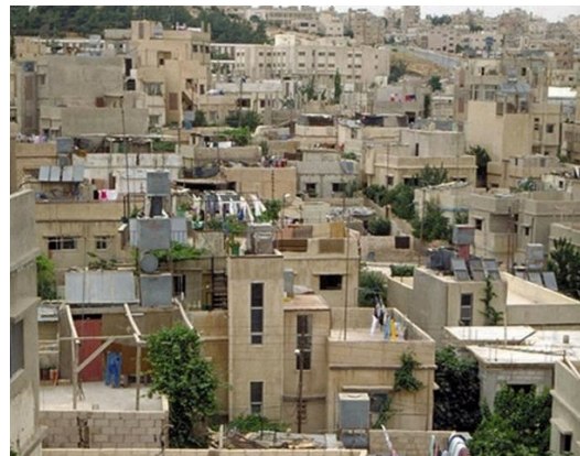
East Wahdat Upgrading Programme, Amman, Jordânia www.archnet.org
