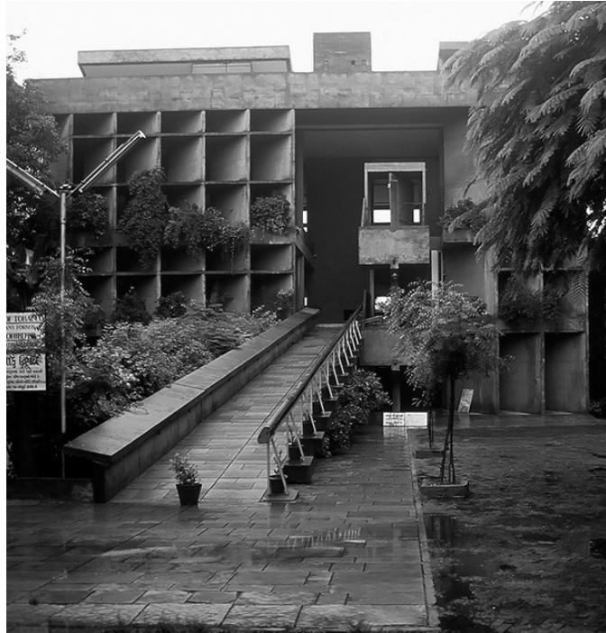
(15) Mill Owners' Association Building (1951) | Ahmedabad, India | Le Corbusier (franco-suíço, 1887-1965)
