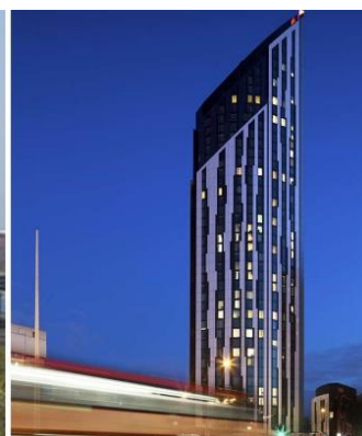
Figura 73. Strata SE1 Tower
