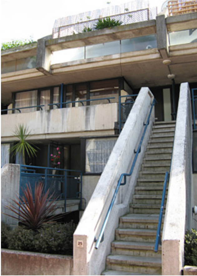
[109] Alexandra Road: Vista Exterior
