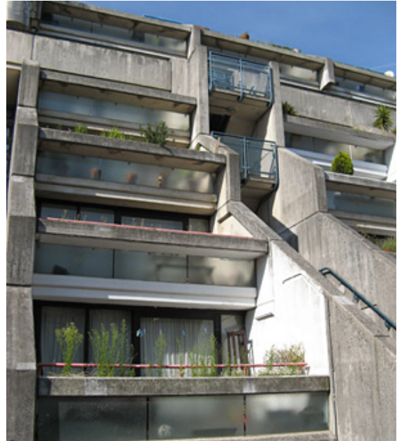
[114] Alexandra Road: Vista Coberturas
