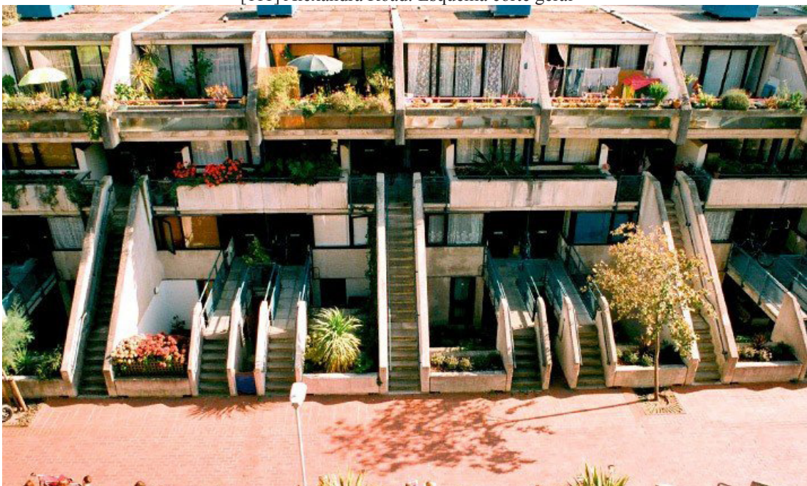
[112] Alexandra Road: Vista Exterior
