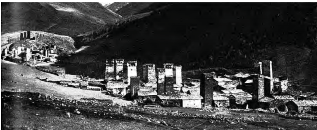
Fig. 7 Bernard Rudofsky, Architecture Without Architects , 1965. As vilas fortificadas de Savetia.
