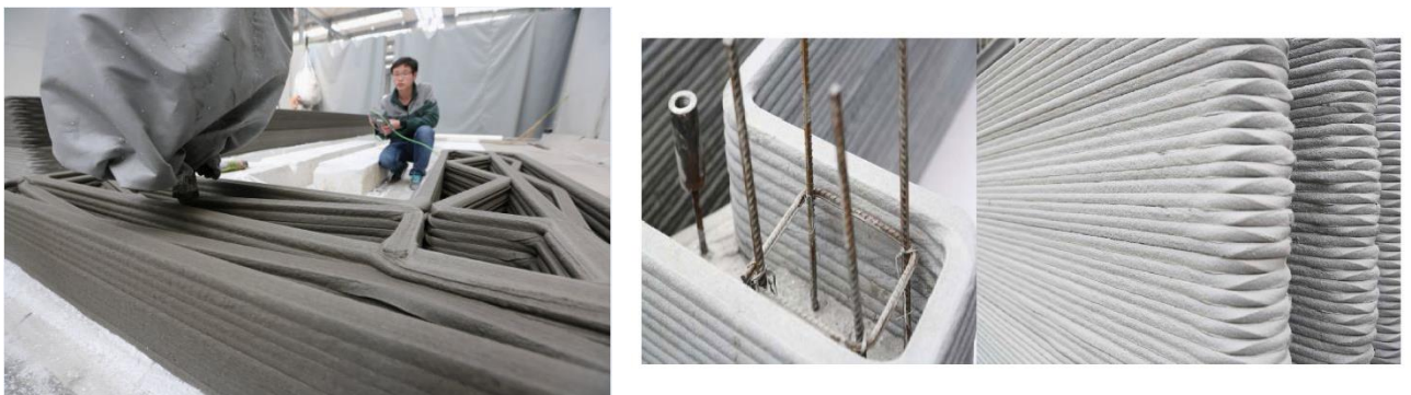
Figure 5.36 – 3D Printed Construction Details [3]
