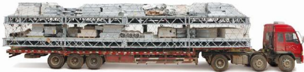
Figure 5.34 – Two 60m 2 modules on a truck [1]
