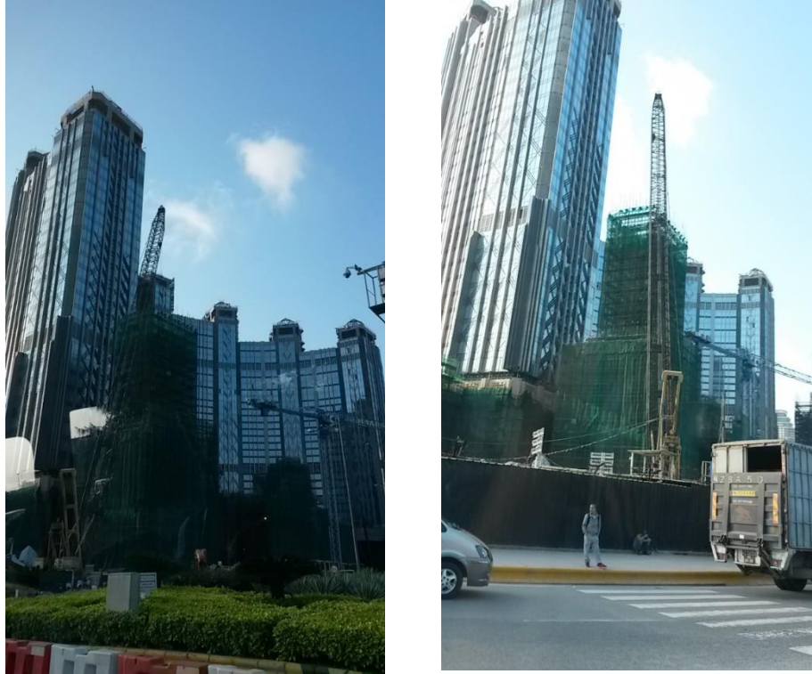
Figure 2.6 – Studio City Construction in Macau
