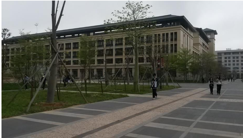
Figure 2.9 – University of Macau Department of Civil and Environmental Engineering
