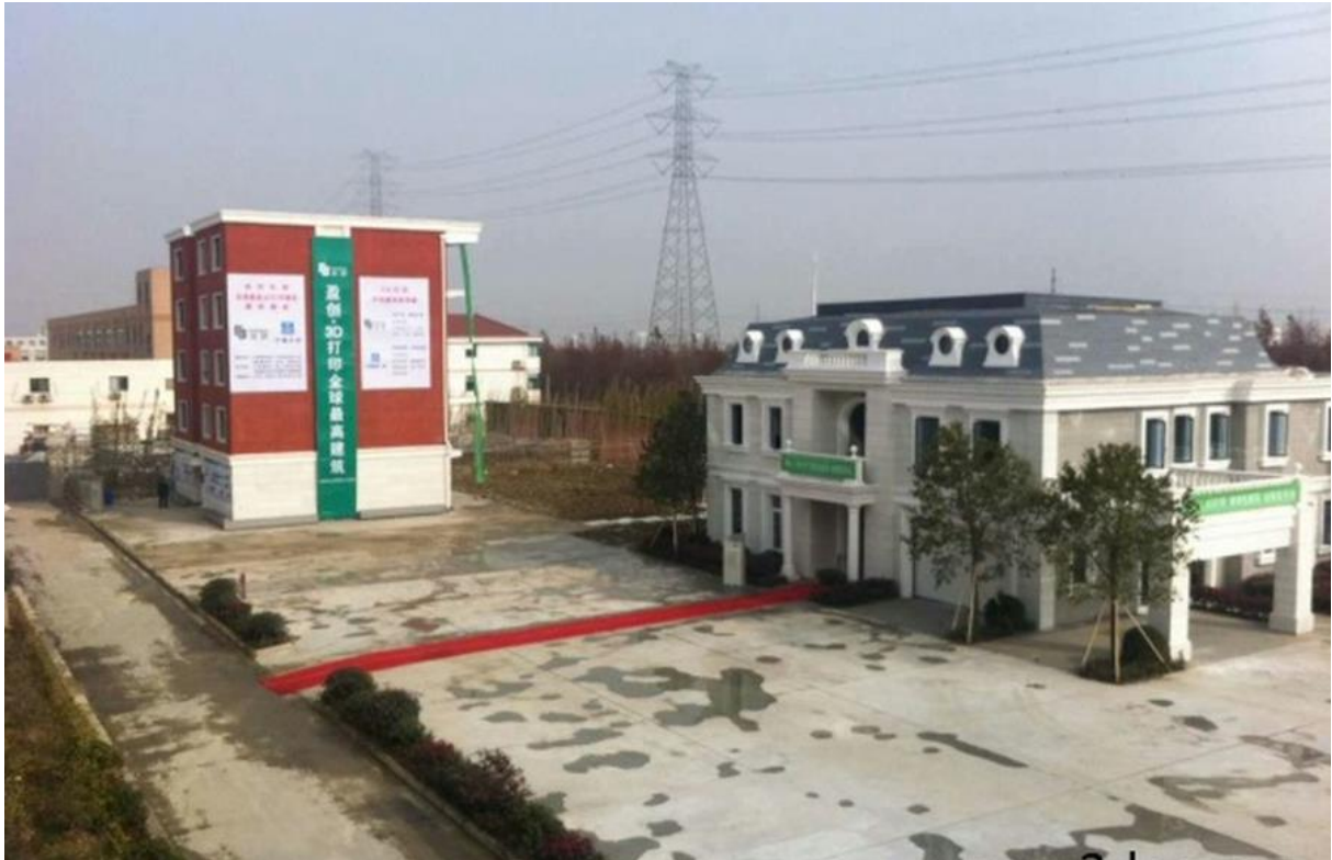
Figure 5.38 – The First 3D printed 5 storey building and Villa by WinSun [3]
