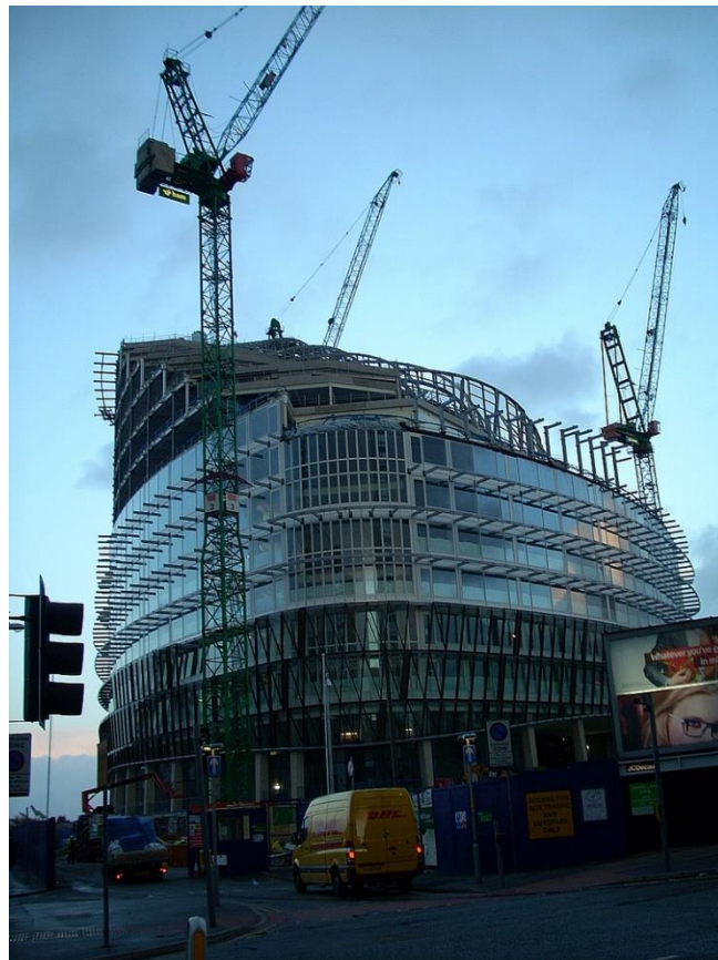
Figure 5.40 – One Angel Square Construction [63]
