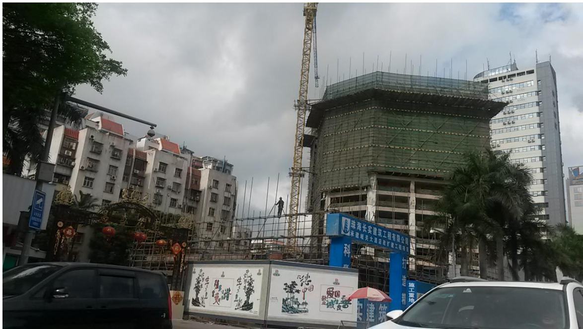
Figure 2.14 – Construction site in Xi'an with bamboo scaffolding
