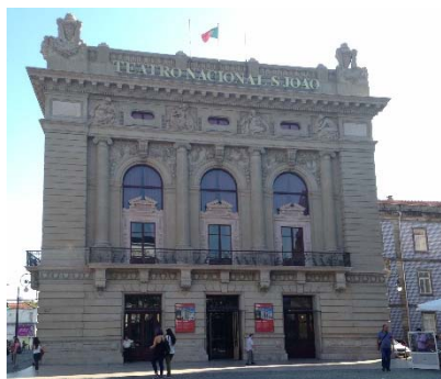
a) Fachada principal
