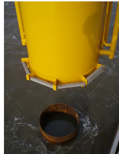
Figure 2- 36: Positioning of the transition piece [38]
