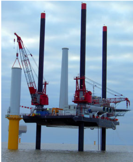
Figure 2- 42: Tower assembled in phases [57]
