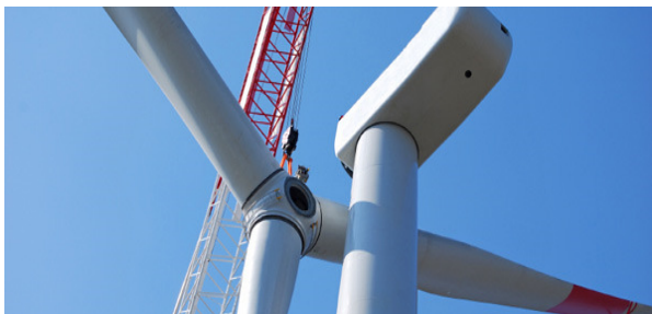
Figure 2- 46: Installation of a pre-assembled hub with three blades [57]
