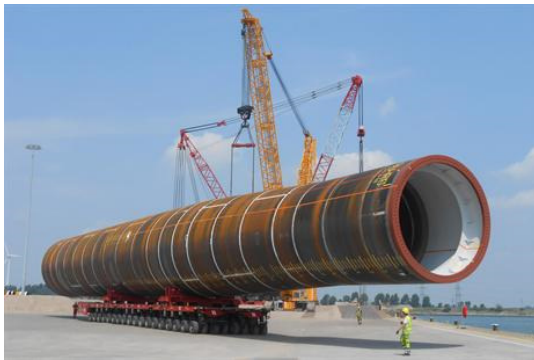
Figure 2- 31: Pile delivered to harbour [38]
