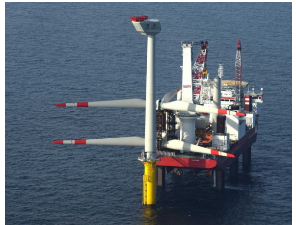
Figure 2- 45: Jack-up barge preparing to install the blades [57]
