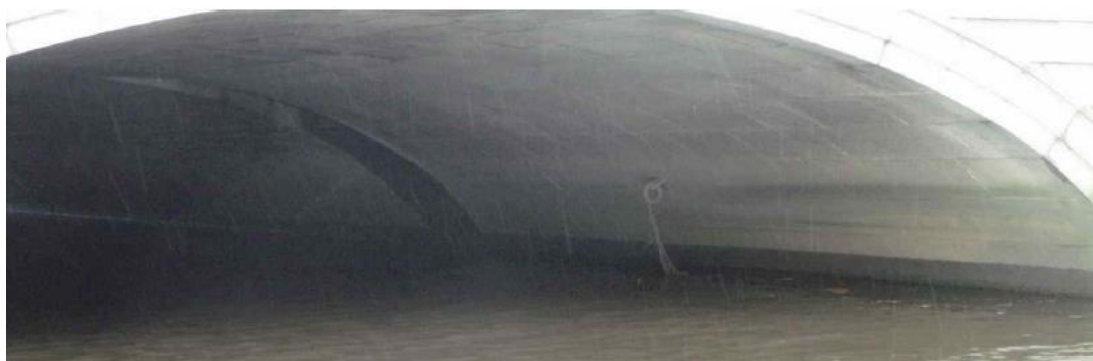
Fig. 108 – Interior do arco [40]
