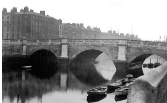
Fig. 97 – Arcos semicirculares de Carlisle Bridge [22]
