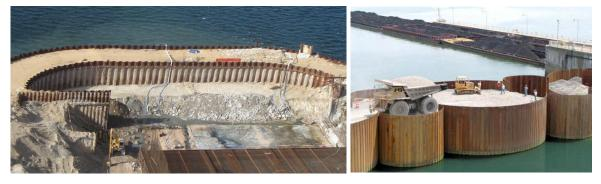
Figure 2.10 - Example of double wall tie cofferdam (left) and cellular cofferdams (right) (C.J. Mahan)
