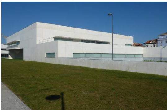
Vista da Fachada Sul Disponível em: http://2.bp.blogspot.com/-pEFw0wZvJJE/TmJWdq87Sol/AAAAAAAAAFE/FRCcItcXN9E/s1600/Biblioteca+Viana+do+Castelo+%25281%2529.JPG
