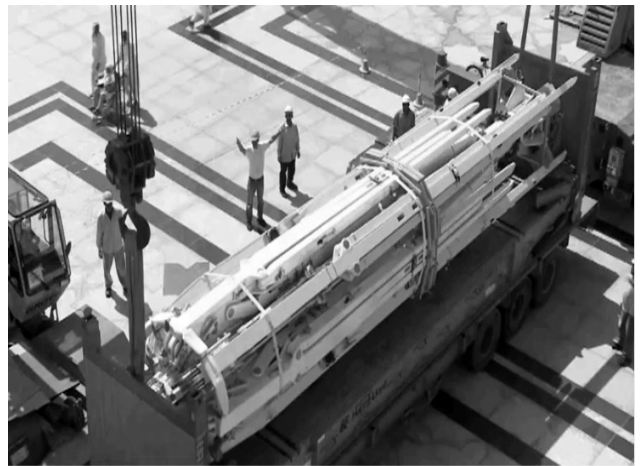
processo de montagem: Umbrellas for the Courts of Prophet's Holy Mosque , Medina, 1992, Frei Otto
