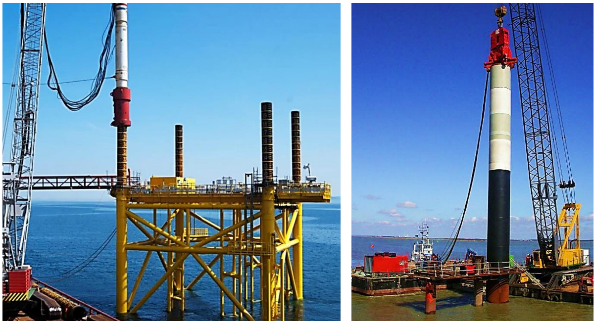
Figure 3.5. – Pile jacking (left) [5]; Vibratory pile driving (right) [6]
