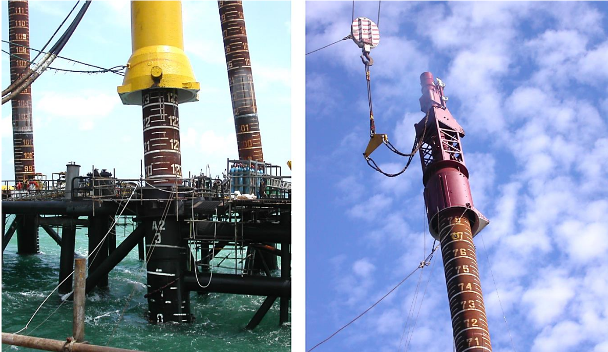
Figure 3.6. – Impact driving process [7]
