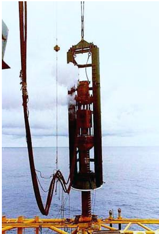
Figure 3.8. – Air/Steam hammer [7]
