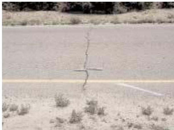
Fig.2.4 - Fenda transversal [13]
