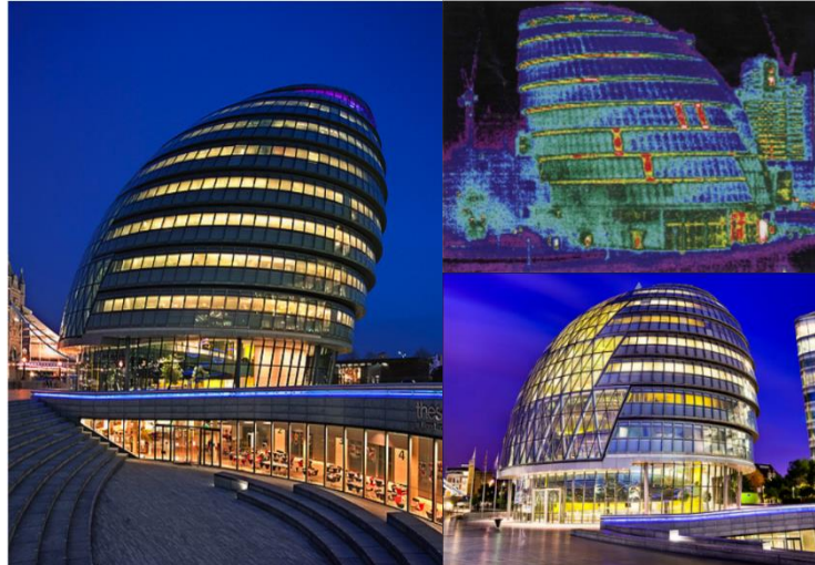
Figura 4.2 - Greater London Authority Headquarters, Londres, Reino Unido, 2002 (Gonzalez, A., 2011).
