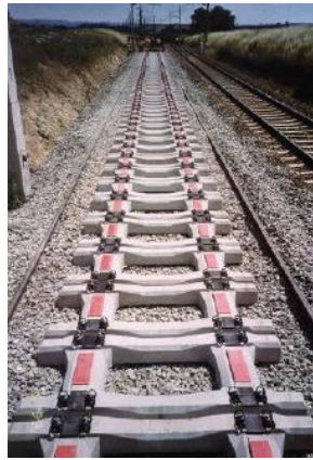
Fig. 4. 7 “Frame Sleepers” (Riessberger, 2006).
