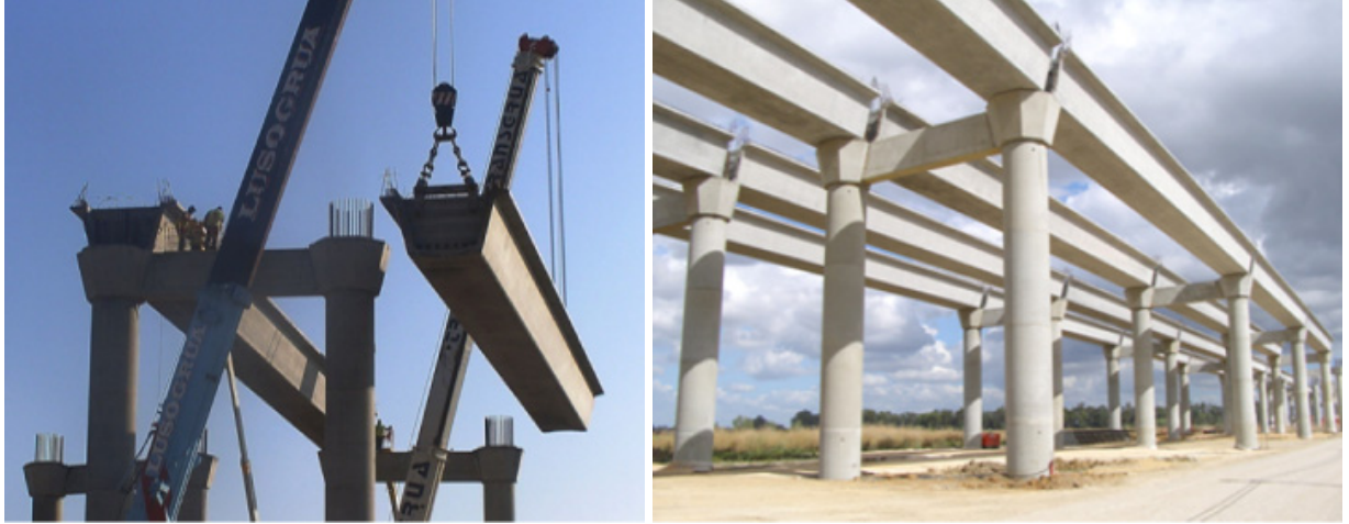
Figure 5.3 – Images of the construction, during the erection of precast girders and before placing the precast planks.
