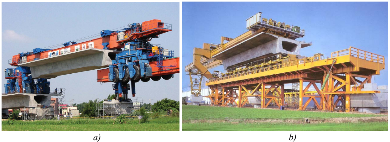
Figure 1.3 – Railway viaducts in Taiwan, each span being made with a single prefabricated element: a) construction with erection equipment by VSL (2010); b) construction with erection equipment designed by Wiecon (2011).
