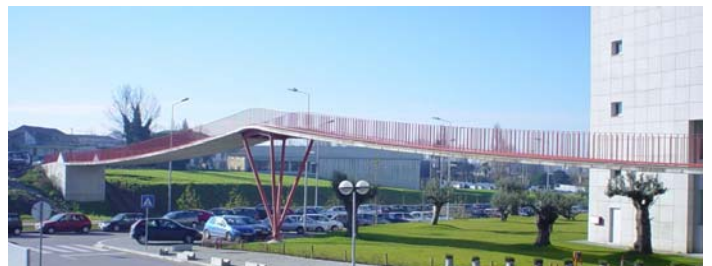
Figure 1. View of the footbridge.
