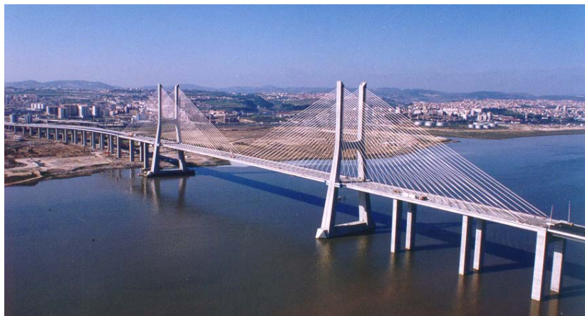
Fig. 1 – Cable-stayed component of Vasco da Gama Bridge
