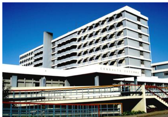
Figura 1 – Hospital da Prelada (SCMP, 2009)
