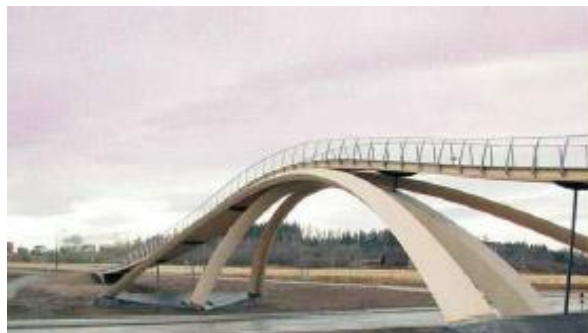
Figure 2: Leonardo Bridge, Aas, Norway.
