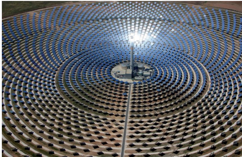
Figure 2.8 Gemasolar Solar Thermal plant using CTR technology with molten salts storage system.
