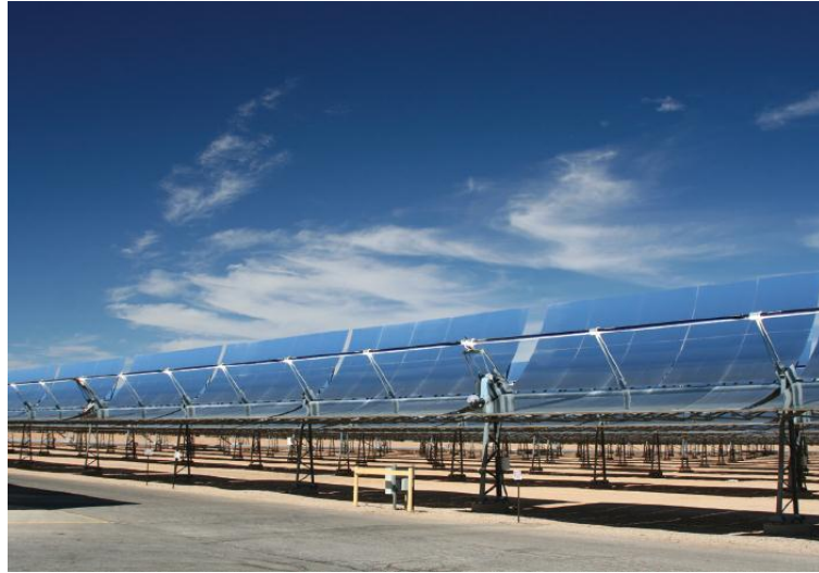
Figure 2.5 Collectors Field of a thermo solar plant with parabolic trough collectors in California (SEGS). Source: (NextEra Energy, Inc., 2012)
