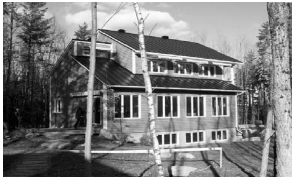
Figure 2.6: The Eco-Terra House, Canada (Noguchi, et al. 2008)
