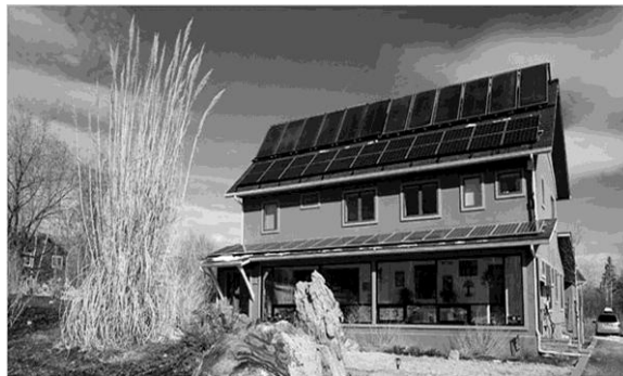
Figure 2.3: Solar Harvest, Boulder, Colorado (Doub, Solar Harvest : City of Boulder ’ s First Zero Energy Home. 2009)
