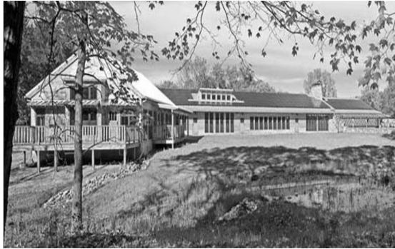
Figure 2.11: The Aldo Leopold Legacy Center, Baraboo, Wisconsin (Thermal Energy Systems Specialists 2007)
