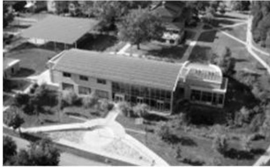
Figure 2.8: The Adam Joseph Lewis Center for Environmental Studies, Ohio (Pless, Torcellini e Petersen, Oberlin College Lewis Center for Environmental Studies: A Low-Energy Academic Building 2004)
