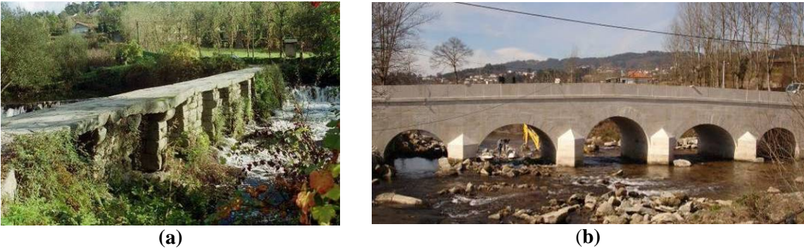
Figure 8: The Vila Fria bridge: (a) old passage and (b) new stone masonry bridge.
