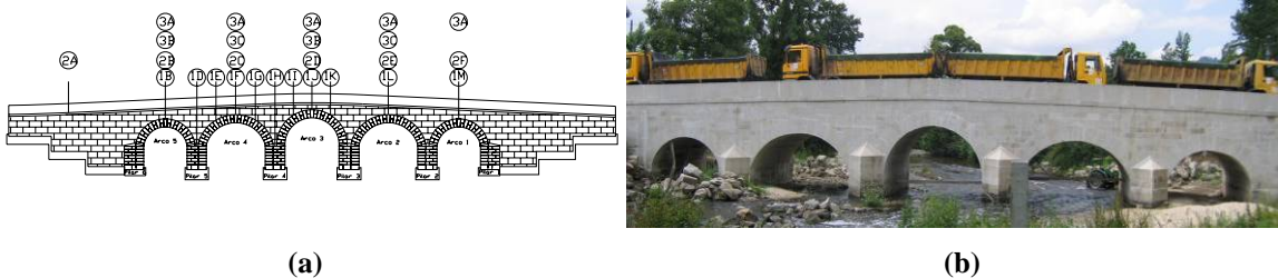
Figure 11: Load test: (a) truck stopping positions and (b) truck arrangement for position 3A.
