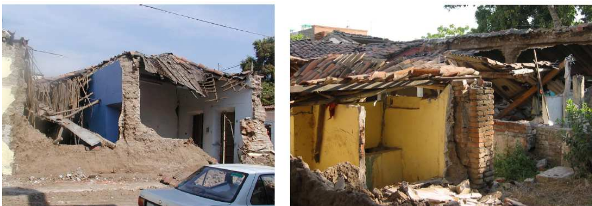
Fig.2.8 – Rotura parcial de casas de Abode [Alcocer, Durán, Flores, Gutiérrez e Reyes, 2003].
