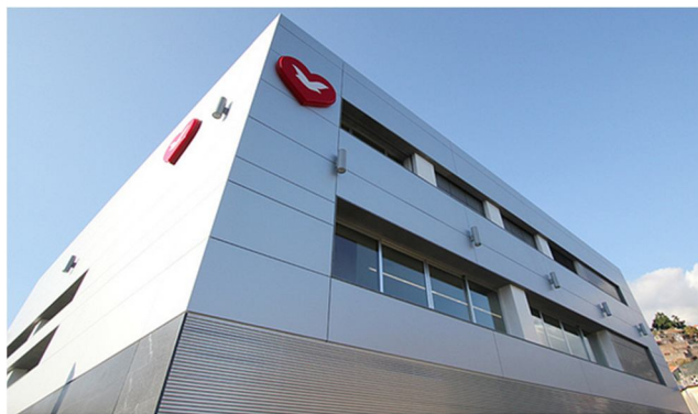
Figura 3.17 – Revestimento de fachada com recurso a alucobond ( http://www.flickr.com/photos/iurdpt/6243969478/in/set-72157627767809641 )
