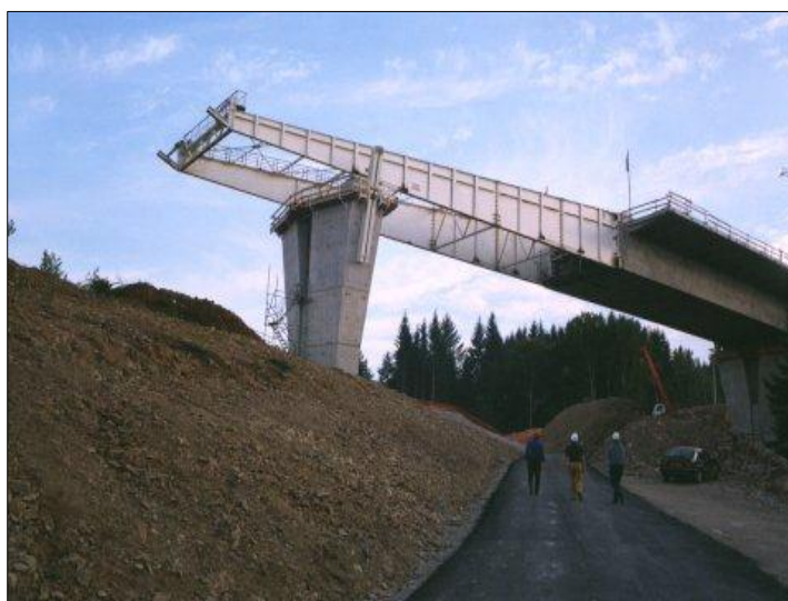
Fig. 2.2.1 – “avant-bec” [2].
