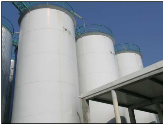
Figura 18. Tanque TK31, TK32 e TK33.
