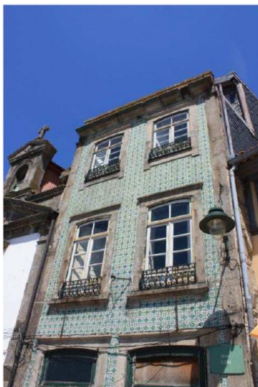
Figura 5.3 – Fachada principal (pisos 0,1,2 e 3)
