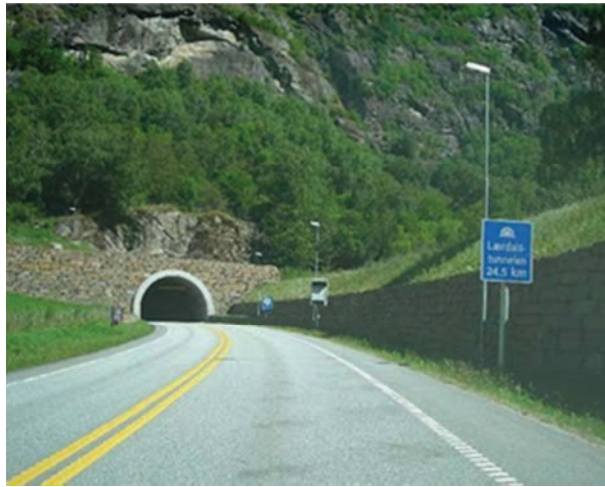
Fig. 1.7 – Túnel Laerdal http://en.wikipedia.org/wiki/L%C3%A6rdal_Tunnel
