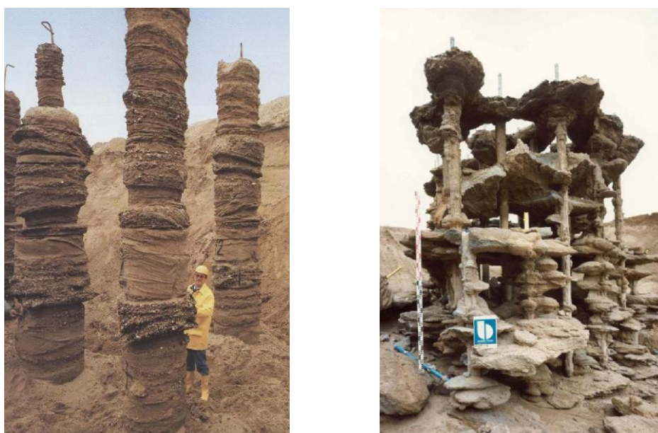
Fig. 3.6 - Colunas de jet grout (Bilfinger, 2010)
