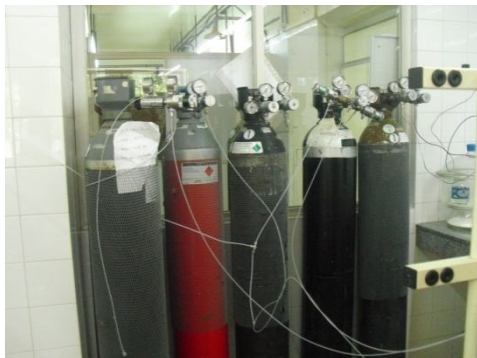
Figure 6: Storage of gas cylinders
