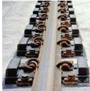
Fig. 14 – Resilient direct fixation fasteners
