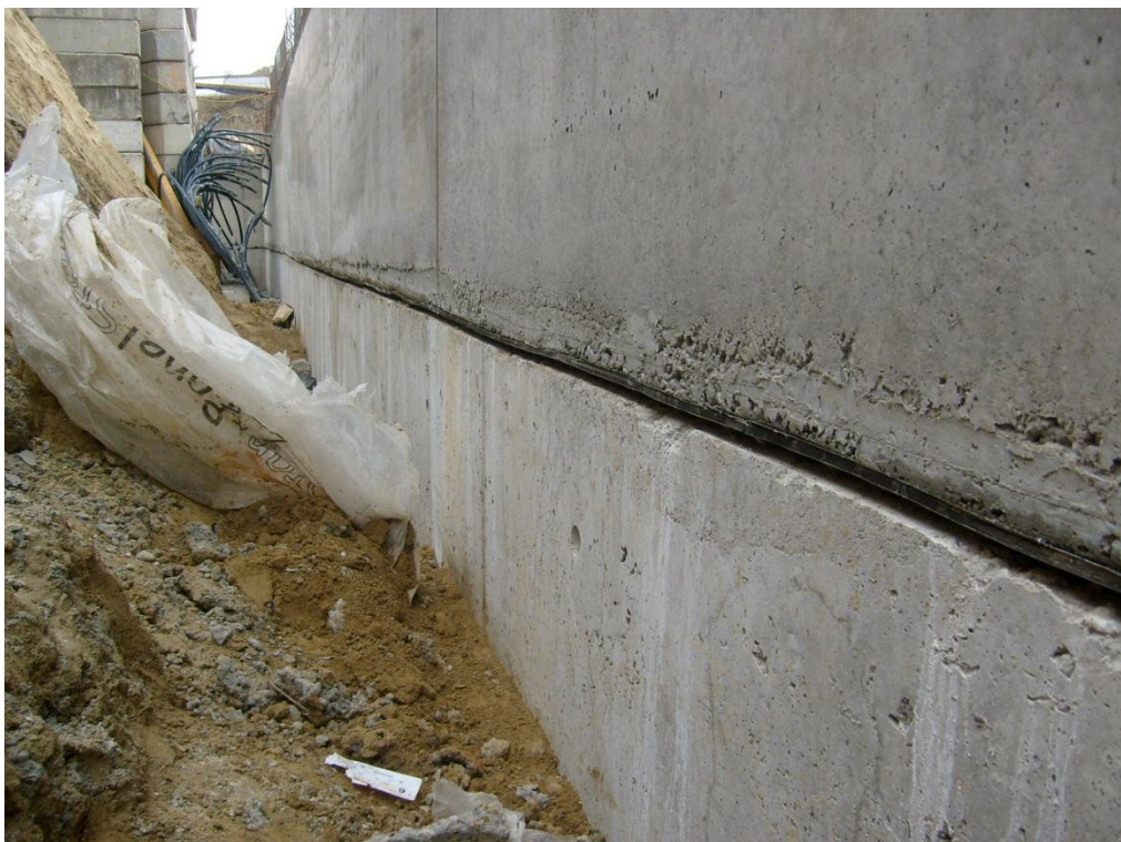
Fig. 22 – Lateral view of bedding elastic for buildings ( iC – Consulanten )
