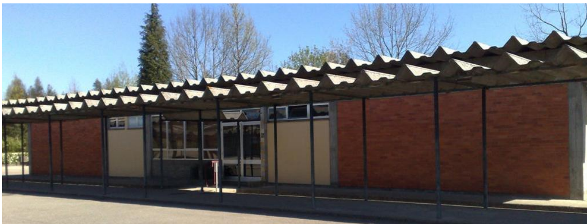
Fig. 11: Fachada principal do bloco (Santos, 2010)
