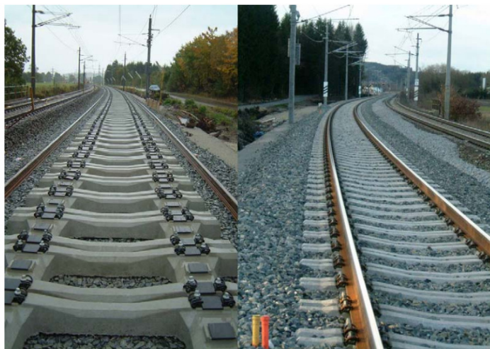
Fig.4. 15 - Travessas "Frame-Sleeper" (Riessberger, 2006)
