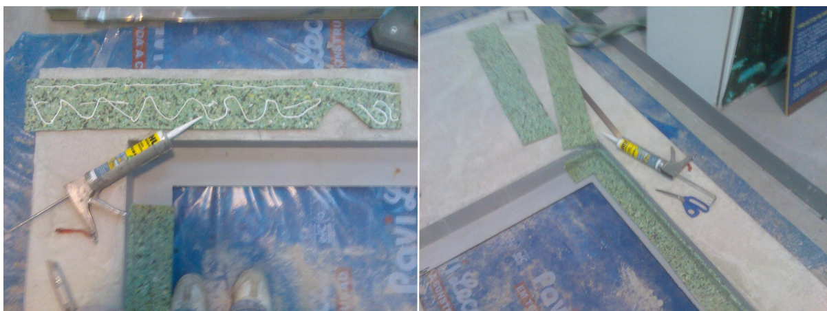
Fig. 4.15: Fitting the base plate opening with the resilient layer
