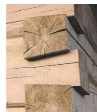
Fig.2.39 – União “Dovetail”
