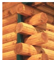
Fig.2.41 – União “Butt-and-pass”
