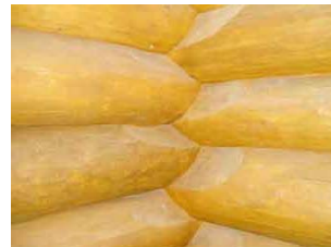
Fig.2.37 – União “Shrink-Fit”
