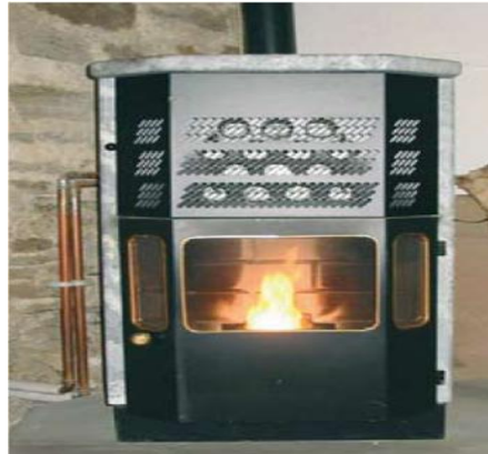
Figure 9: Biomass boiler (pellet stove with back boiler).
