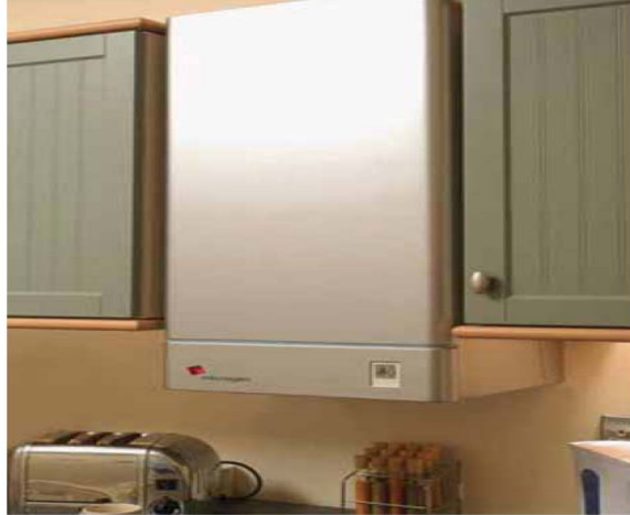
Figure 10: Wall mounted micro-CHP system installed in kitchen.
