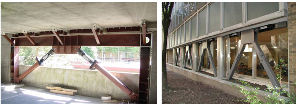
Fig. 2 – a) Amortecedor Viscoso [12]; b) Portland State University [13]
